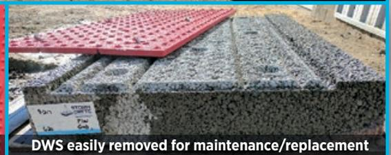
DWS easily removed for maintenance/replacement
